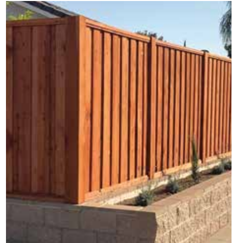
INSTALLED LIFEPOST APPLICATION
