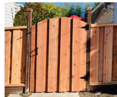
Board on Board Nail on Arched Gate
