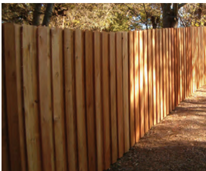
Board on Board Nail On
