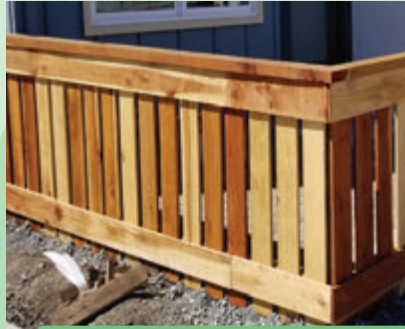
● Gap Style Nail On with 1x4 fascia top and bottom and 2x6 cap
