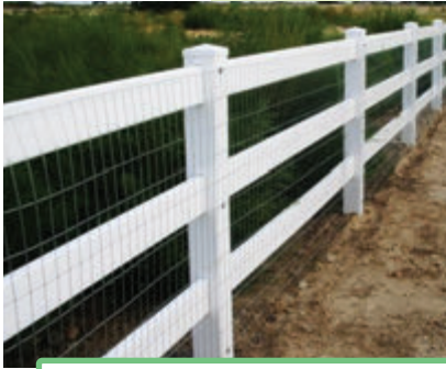
● Wire on Existing Fence
